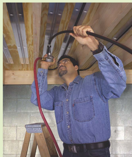
Climate Trak grips the company's tubing to prevent air gaps or loss of direct contact between the tubing and the snap channel.
