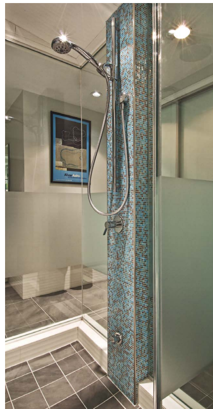
The mosaic tiled "shower tower" was a solution for moving the plumbing off the exterior wall to avoid frozen pipes in winter.
